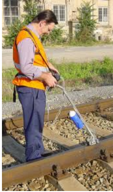
(a) An ultrasonic flaw detector with a combined probe for manual inspection
